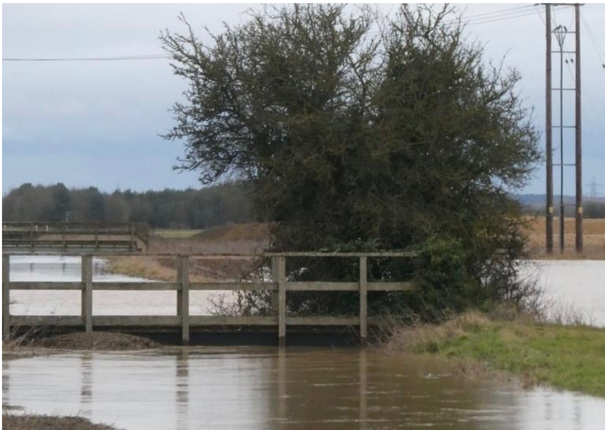
Figure 6.1 – Flood conditions during 2024. View looking north along the drainage dyke opposite the proposed Baston Green development site. Water is visibly extending around the bridge structure and beyond the apparent normal confines of the drainage channel into the surrounding land.
